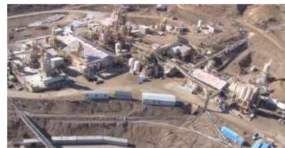
Exhibit 2: MP Material's processing facility operated in the mountain pass mine located in the Clark Valley Range in California.
